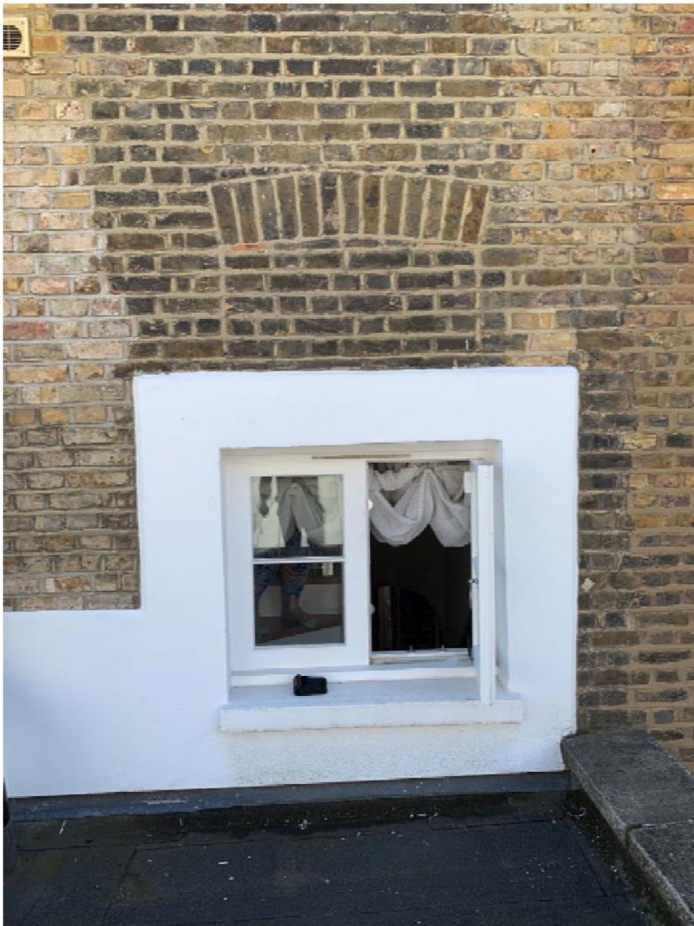
Existing first floor window
